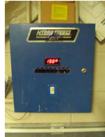
Original step controller used to match performance of boiler plant with outside air and return water temperature inputs
