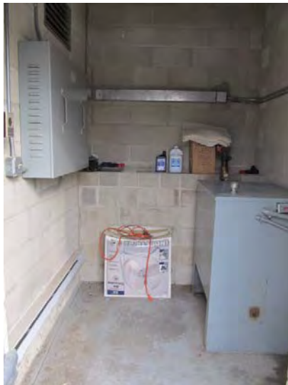
Controller/dispatcher and hydro-mechanical unit for elevator maintained under terms of a full service contract – No near-term needs anticipated
