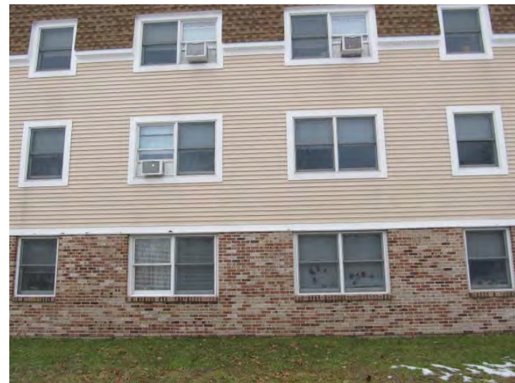
Vinyl siding and mansard shingles replaced in recent years and in good condition – Original windows typical throughout building
