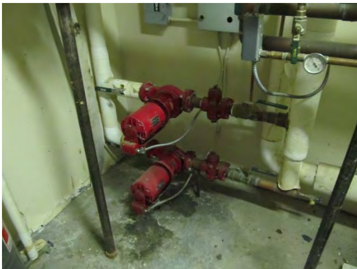
Inline pumps for circulation of hydronic heat to common areas and dwelling units
