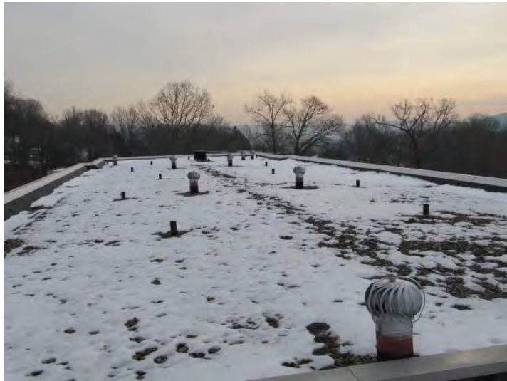
Ballasted membrane coverings on flat roof surfaces are in generally good condition for their age
