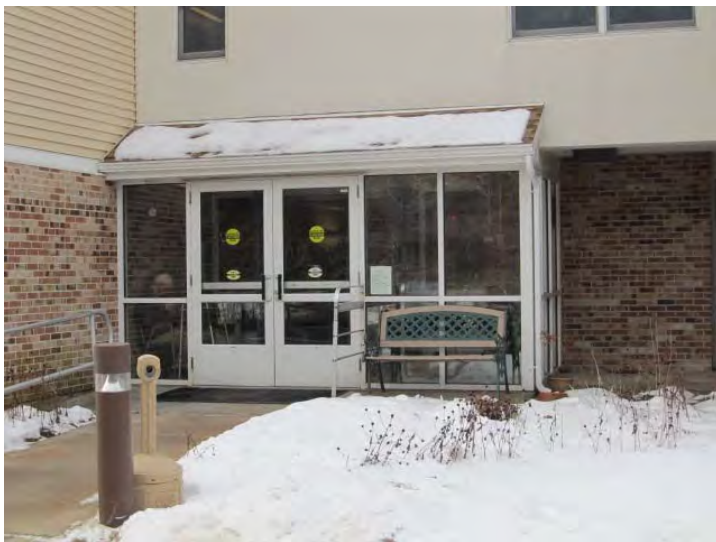
Aluminum and glass doors at main entry to building are in good condition
