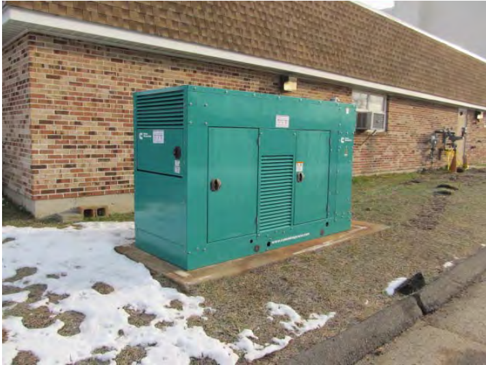
Installation of new Onan natural gas-fired generator for emergency power nearing completion at time of assessment
