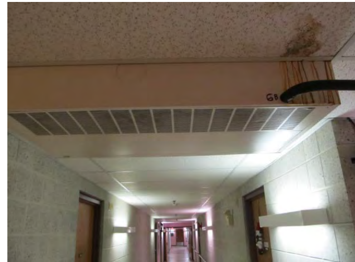
Typical ceiling-mounted fan coil component for cooling of common hallway
