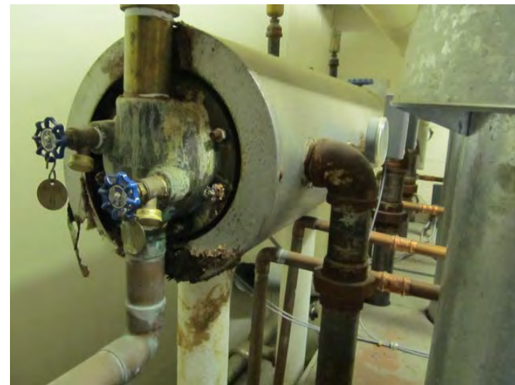
Shell and tube heat exchanger for production of domestic hot water – Note rust/deterioration at bottom of unit
