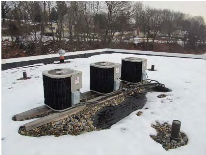
Three of six rooftop-mounted, air-cooled, condensers used to provide air conditioning to common hallways
