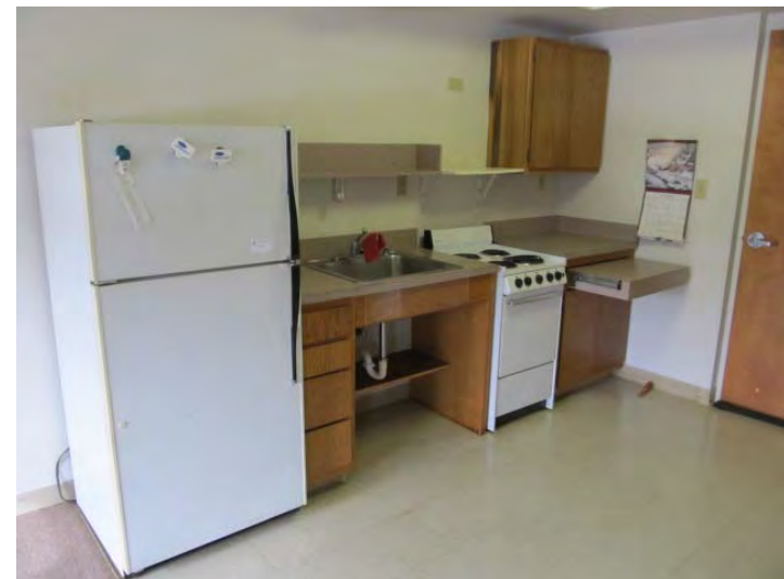
Countertop at handicap accessible unit kitchens exceeds height limits, work surface is too small, and piping under sink lacks insulation
