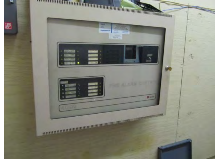
Original zone-type fire alarm control panel
