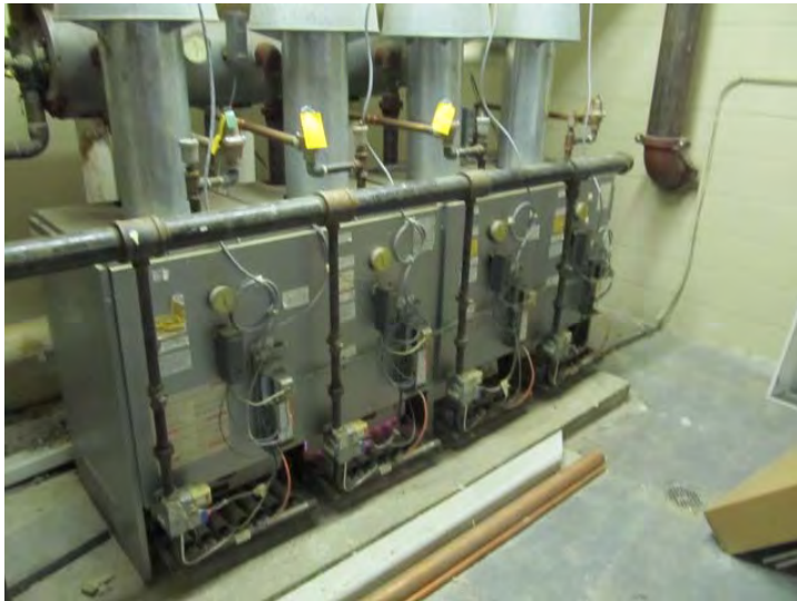
Original, natural gas-fired, modular boiler plant produces hydronic heat for distribution throughout the building
