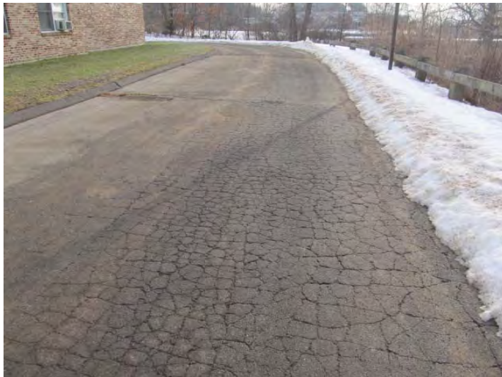
Cracks and wear evident noted at asphalt service drive along rear elevation of building
